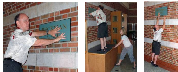
Figure 1 (a) (b) and (c): Signage, which incorporates Braille, but does not take into account accessibility resulting in problems for the intended user
