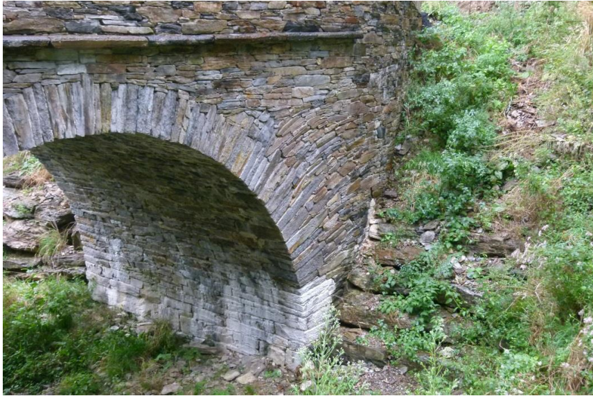
Figure 3: Focus on the haunches of Chaldecoste Bridge (Photo credit: P. Mc Combie)
