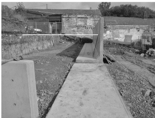
Figure 2: The site at the start of the construction phase.
