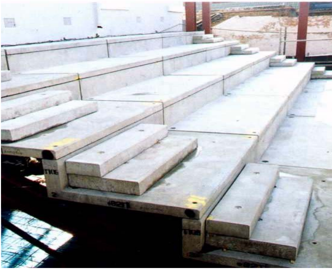
Figure 1 Precast concrete terraces.
