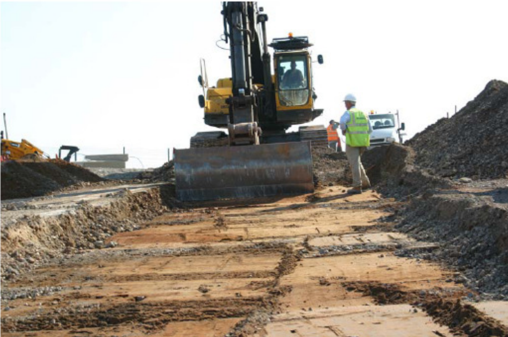
Figure 100. Trimming and levelling the trial area to expose the sub-grade.
