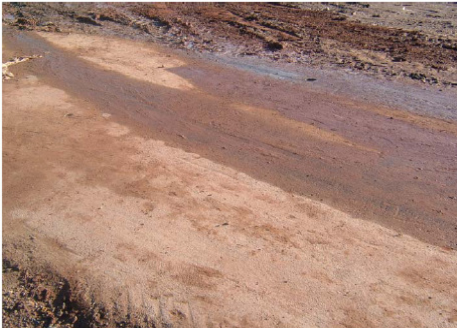
Figure 122. Close-up of the trial road at the King's Mill Hospital site.
