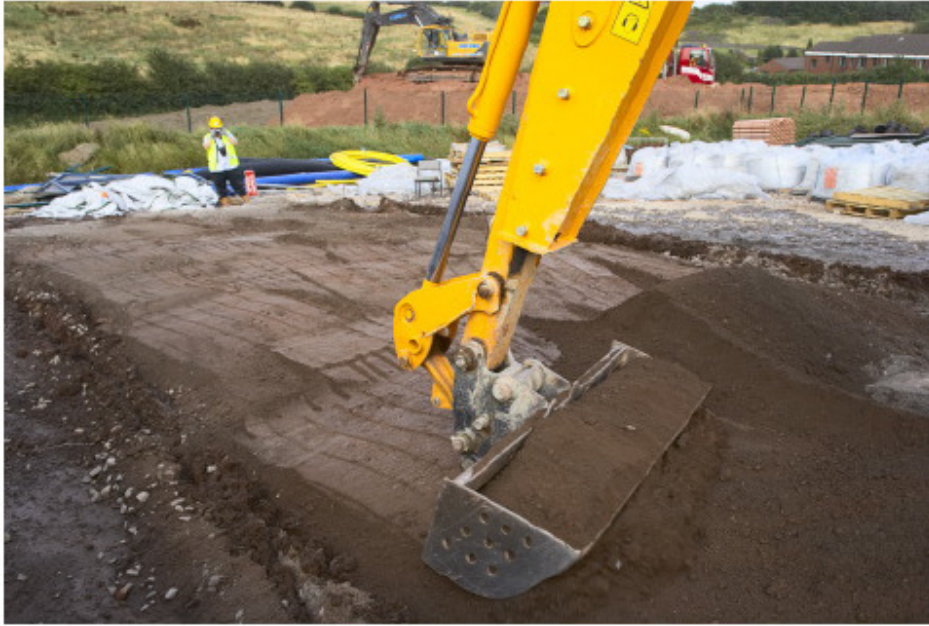
Figure 110. Levelled blended soil and powder ready for compaction.
