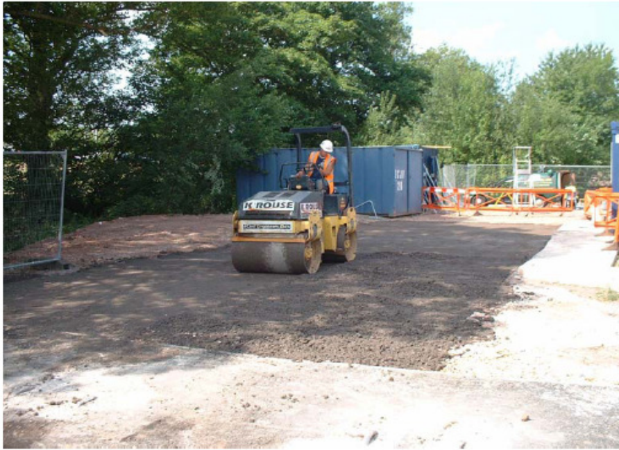
Figure 95. Concrete compaction using a 3-tonne vibrating roller.
