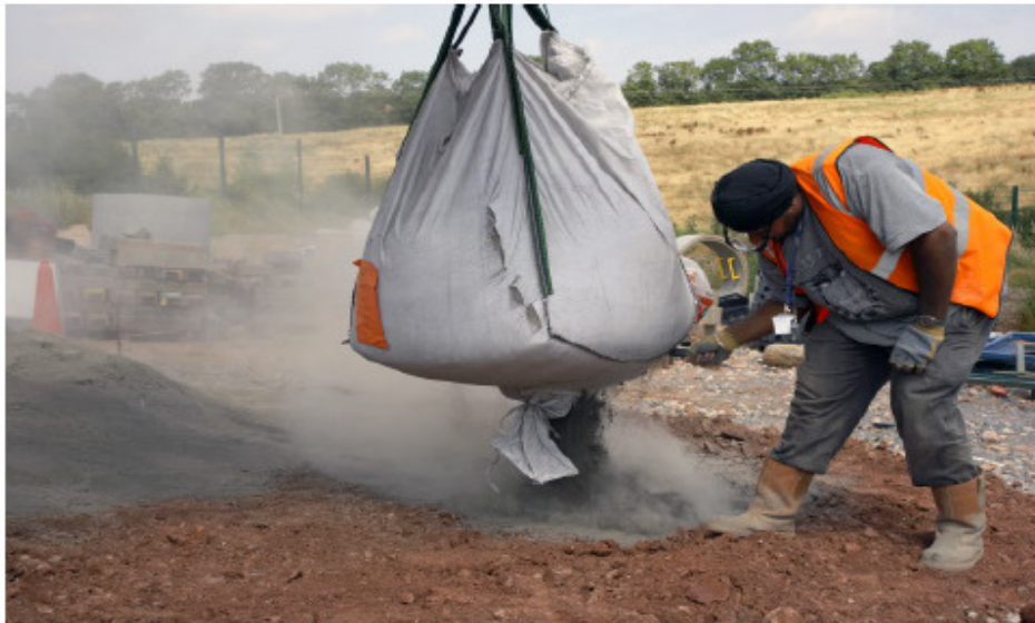
Figure 104. Placing and spreading the powder on top of levelled soil.
