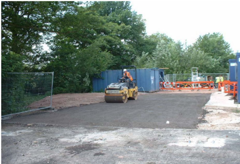
Figure 96. Completed 100-mm layer of RCC at the Lowdham Grange site.
