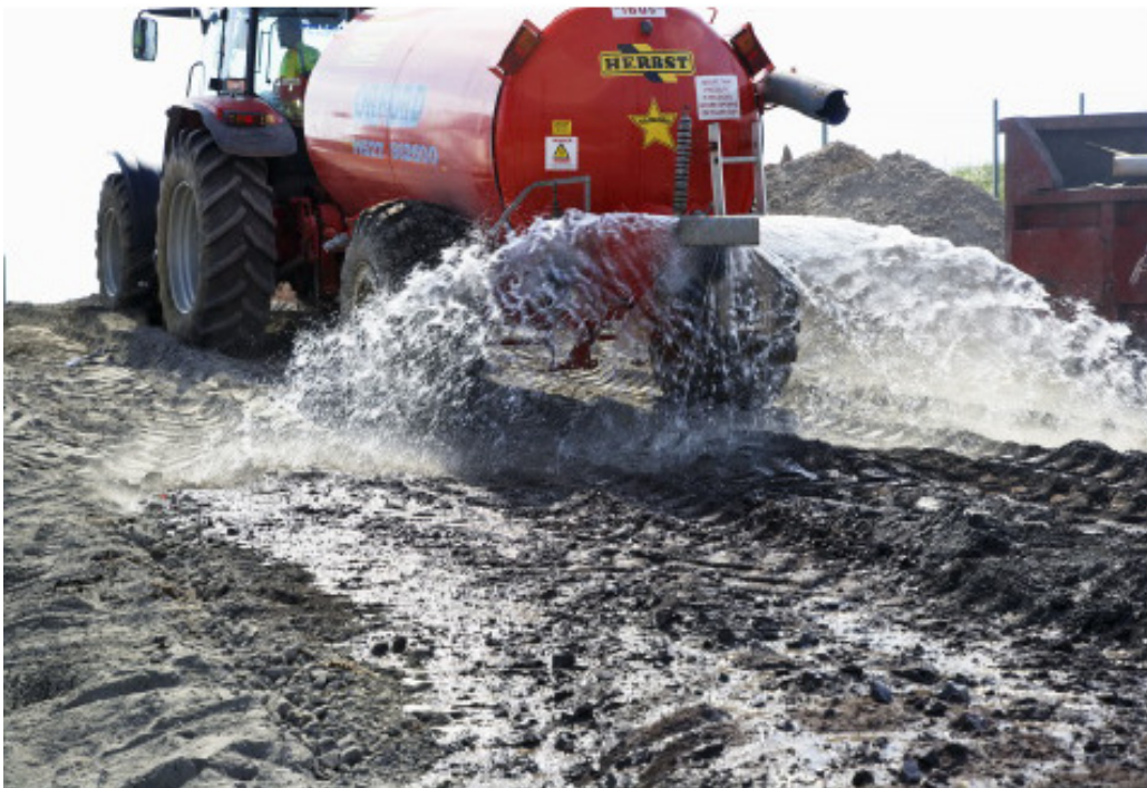
Figure 109. Watering the mixture of soil and the binder using the sprinkler.
