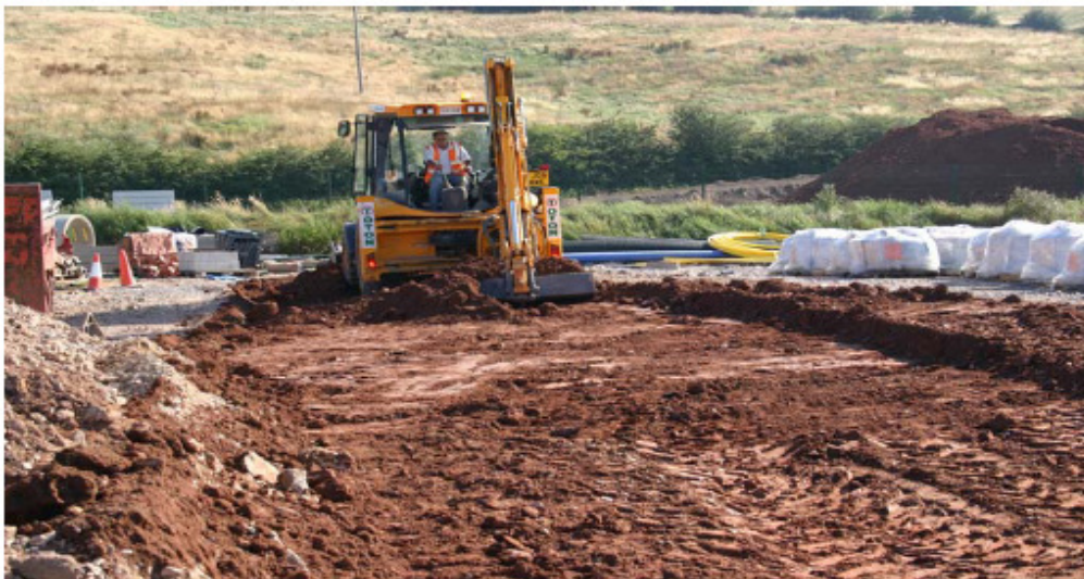
Figure 102. Levelling the spread soil using the JCB.
