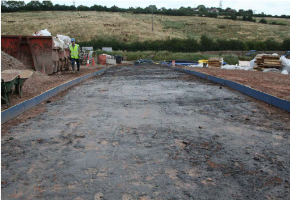
Figure 114. Sprayed surface of stabilised soil before constructing the paste layer.
