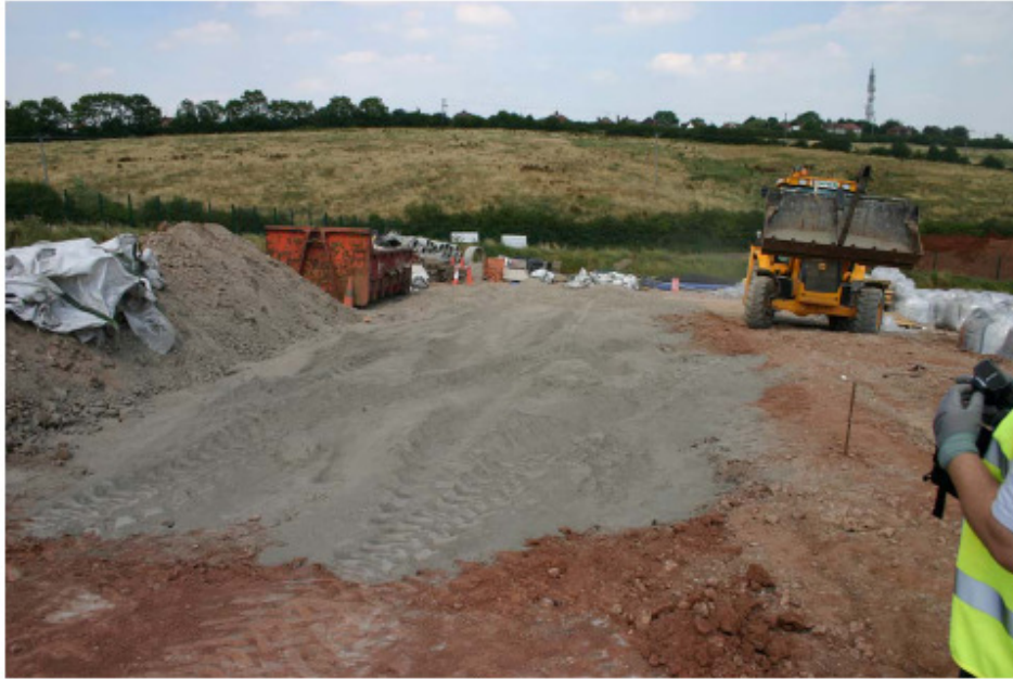
Figure 105. Levelled layer of powder on top of the soil.
