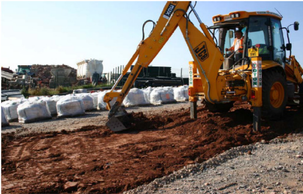
Figure 101. Spreading and levelling the soil in the trial area.
