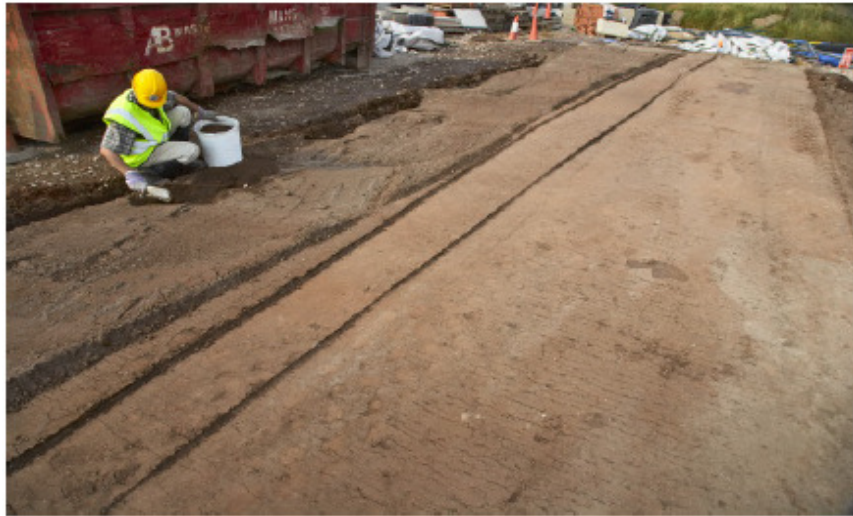
Figure 112. Finished surface of the stabilised soil.
