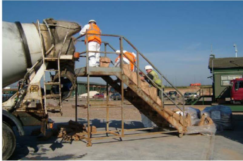
Figure 90. Loading blended binder into the truck mixer.
