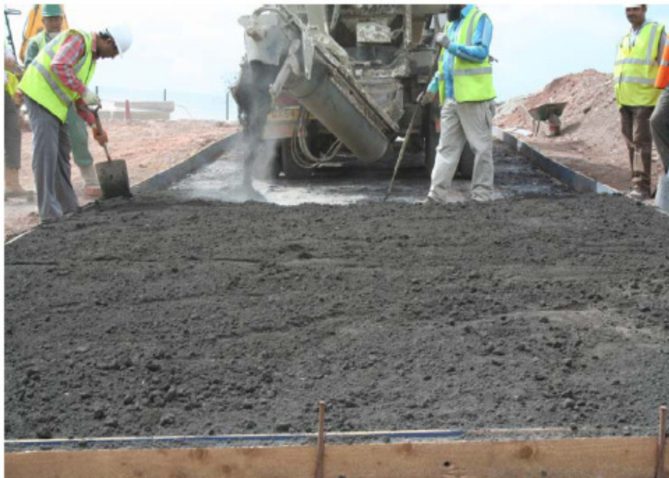
Figure 116. Spreading and levelling the semi-dry paste.
