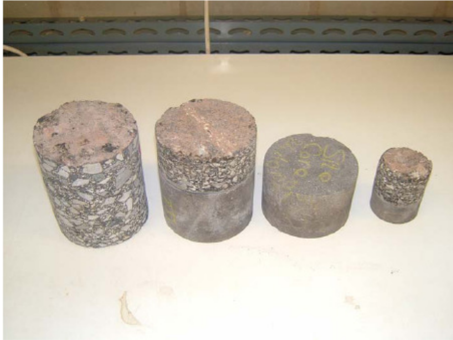
Figure 125. Core samples taken from different locations in the trial road at the King's Mill Hospital site.
