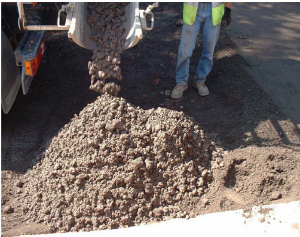
Figure 92. Placing concrete using the truck mixer chute.
