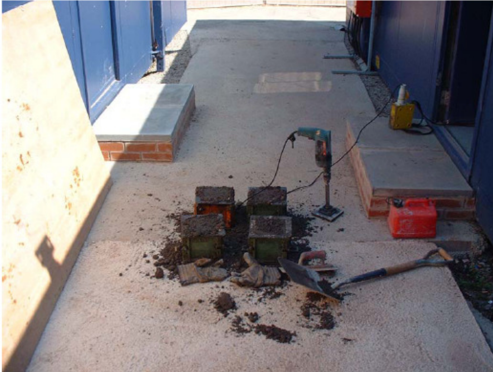
Figure 97. Sampling of concrete using 150-mm cubes and hammer drill.
