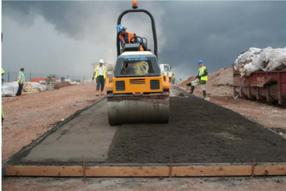
Figure 117. Compacting the semi-dry paste layer using a 3-tonne roller.
