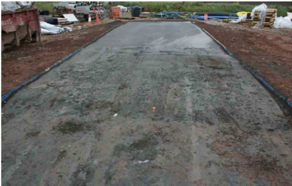
Figure 118. Finished surface of the compacted semi-dry paste.
