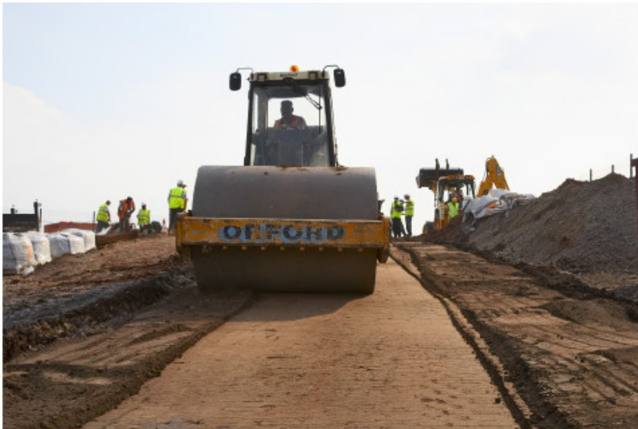
Figure 111. Compacting the blended soil and the binder using the 10-tonne roller.
