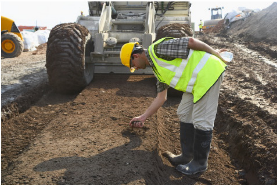
Figure 108. Inspecting the blended soil and powder before adding extra water.
