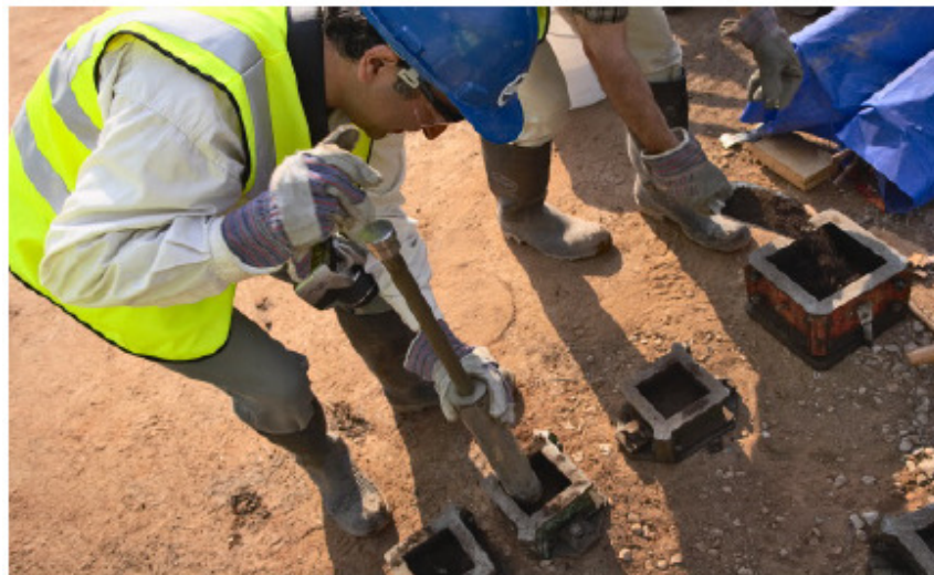
Figure 113. Sampling the stabilised soil.
