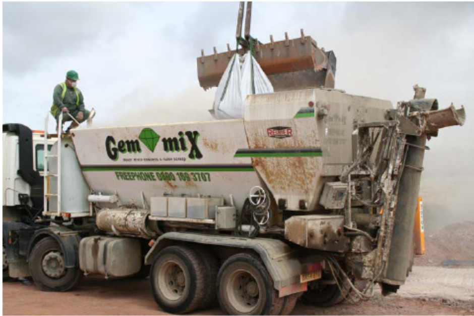
Figure 115. Loading the mixer with blended powder.
