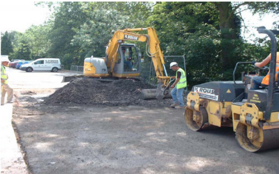
Figure 94. Spreading the concrete using a mechanical excavator.
