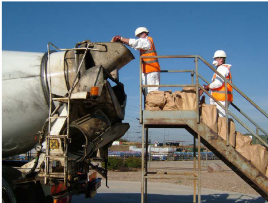
Figure 91. Loading blended binder bags into the truck mixer.
