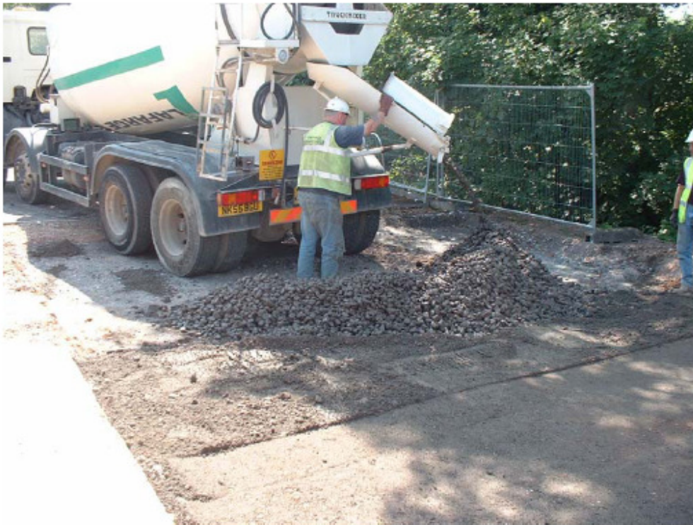
Figure 93. Placing and spreading the last batch of concrete.
