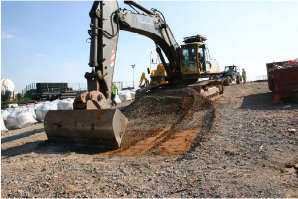
Figure 99. Preparation of the trial area using an excavator.
