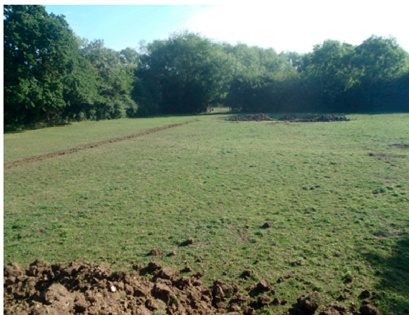
Figure 1. The compacted horse grazing field, prior to installation of the Wetland Ecosystem Treatment System.
