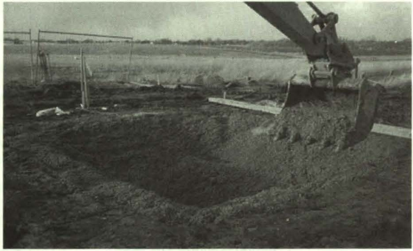
Fig. 3. Placing concrete in the field trial
