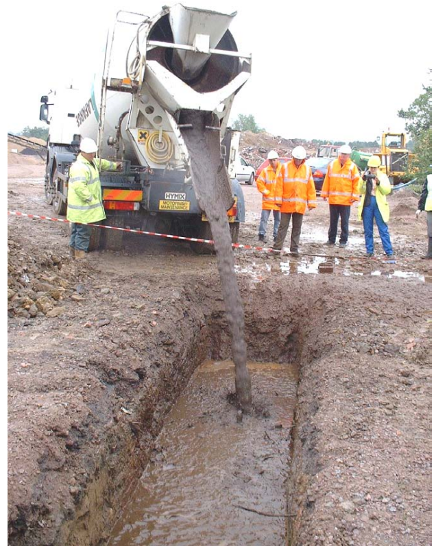
Fig. (19). CLSM Discharge to trench.
