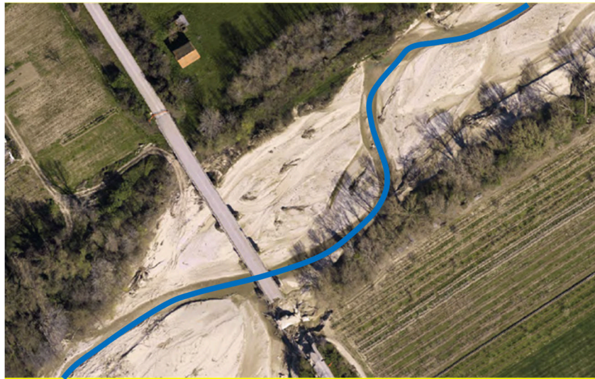
Figure 3. Path of the meandering Aso river in 2015 (a few months before the collapse of piers n. 4 and n. 5).
