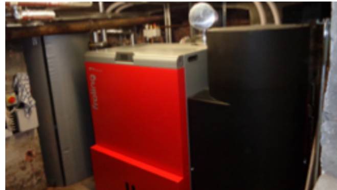
Figure 6 – Gwent Energy installed 100 kW biomass boiler at Wellington Baptist church and community centre (Gwent Energy CIC, 2019c)
