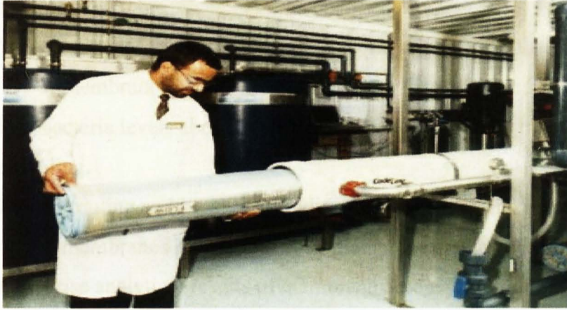
Figure 2.25: Removal of membrane element, (Darton and Faxell, 2001).
