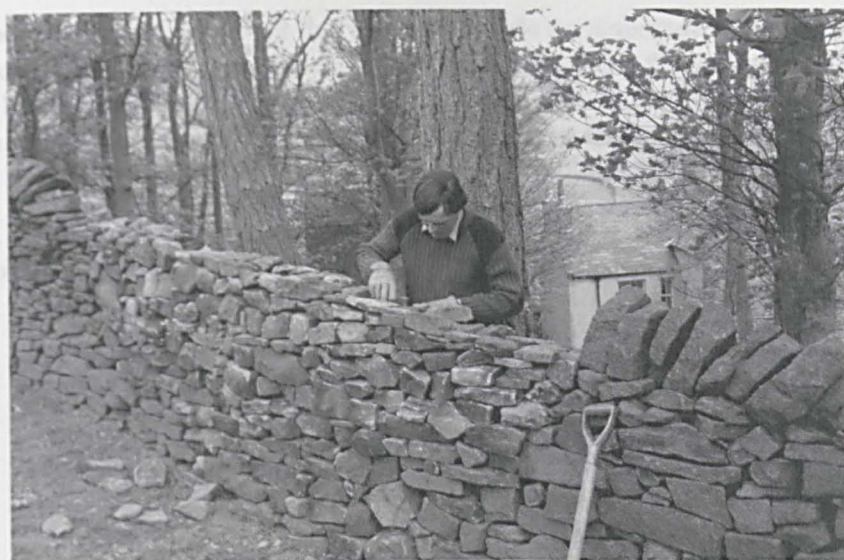
Photograph 9.13. Rebuilding a field wall in the Upper Derwent. National Trust Collection
