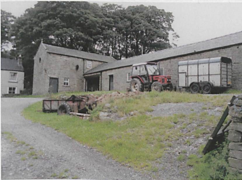
Photograph 7.9. Estate style barn architecture dating from the 19 th century at Blackden View, Hope Woodlands
