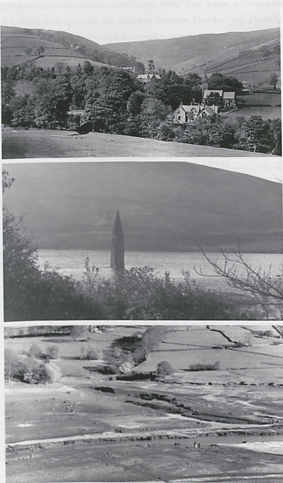
Photograph 8.17. Three views of Derwent Village in the 20 th century. Looking from the west in the 1920s (top), looking from the east when only the church spire remains above water in the 1940s (middle) and looking from the west again - the ruins lie exposed on the bed of Ladybower Reservoir in 1995. PDNPA Collection
