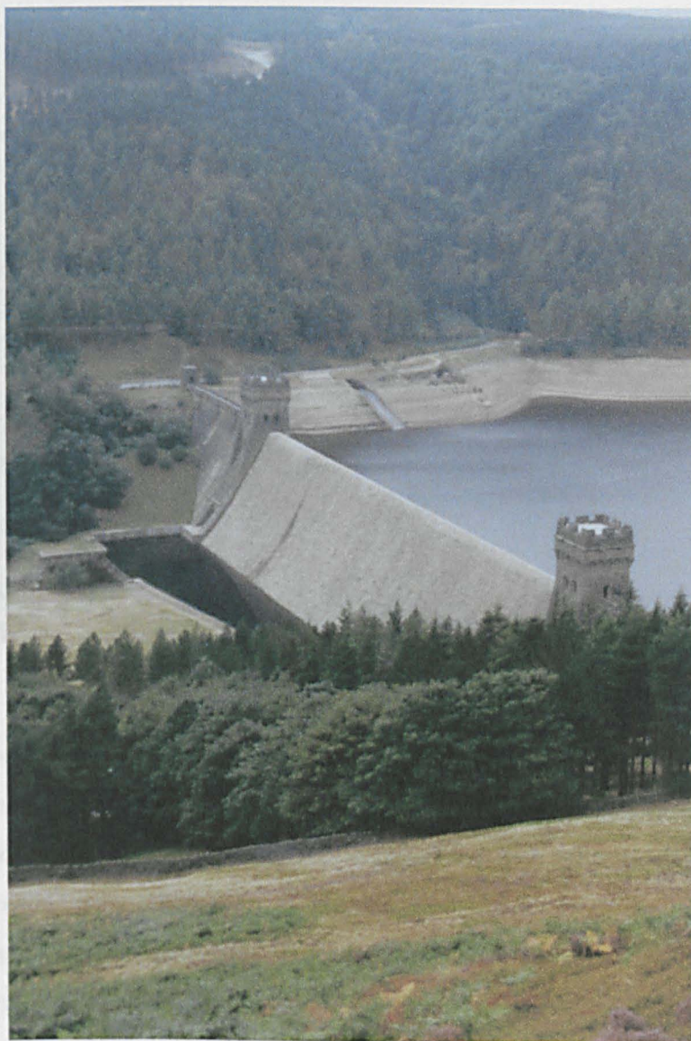
Photograph 8.1. Derwent dam, looking north-west
