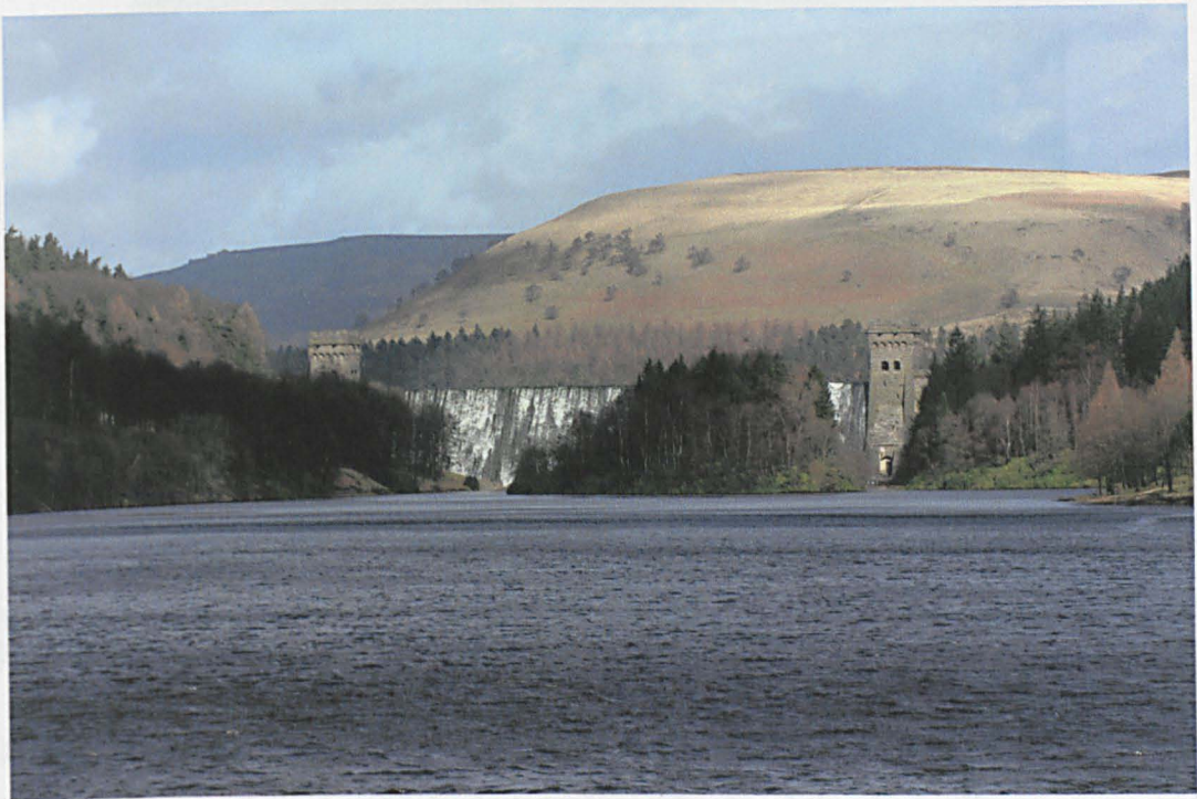
Photograph 8.2. Howden dam, looking north. PDNPA Collection
