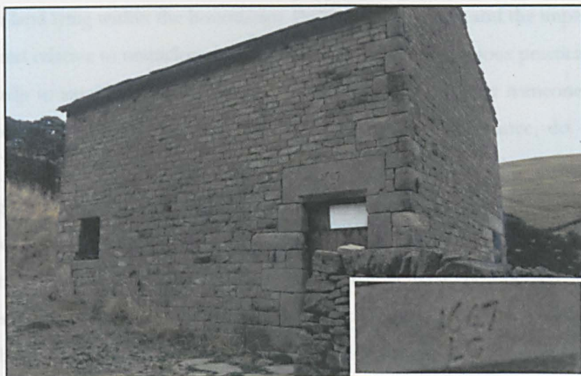
Photograph 6.3. Field barn at Grindle Clough, with dated lintel inscribed 1647
