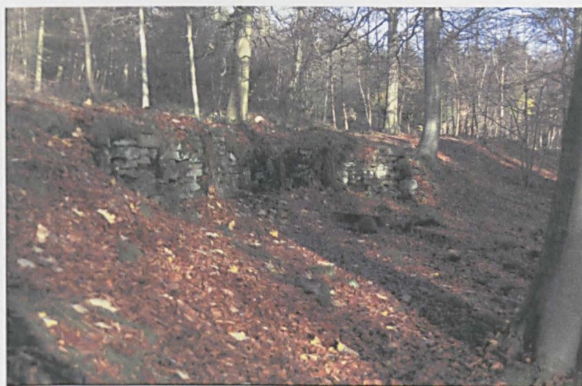
Photograph 8.13. Stone revetted platforms for the outside toilets at Tin Town
