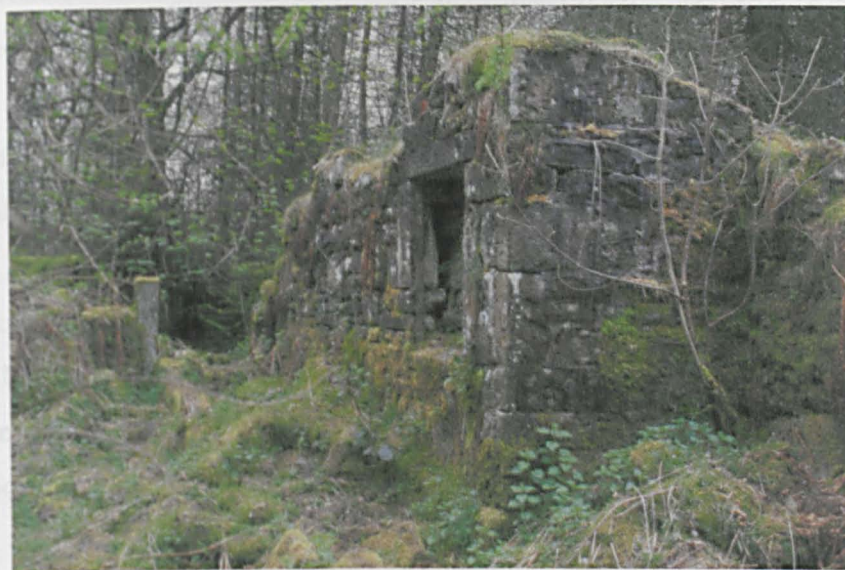
Photograph 9.12. Elmin Pitts farmstead. Elmin Pitts is one of only five farmsteads abandoned during the creation of the three reservoirs where substantial building fabric was left standing by DVWB. Like many of the farmstead sites it now survives within a woodland with public access managed by Severn Trent Water. Conifers around many of the ruined farmsteads are being clear-felled to prevent further damage from forestry activity, but the woodland around Elmin Pitts will be left in place because it mainly comprises deciduous species with a high wildlife habitat value
