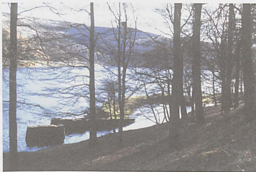
Photograph 8.4. Bridge supports for the Bamford and Howden Railway
