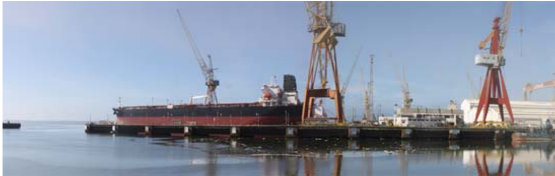
Figure 1 - View of the Quay 3.
