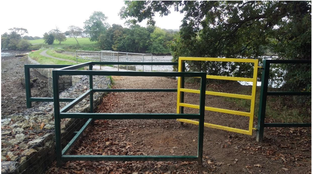
Figure 7.8 Kissing gates installed along Headland Path at Ernesettle, September 2017
