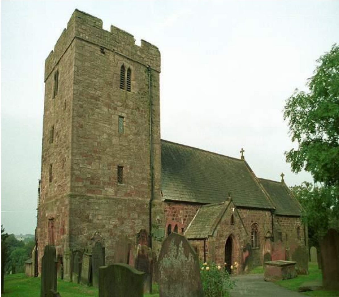
Figure 5: Dearham Church, North West Cumbria, is an example of a church with fortified tower of 12 th Century origin date (Historic England 2018). The image conveys the structural sturdiness and practicality of the tower, with small windows in each storey and no entrance directly into the tower, except through the church itself (picture Visit Cumbria 2018).
