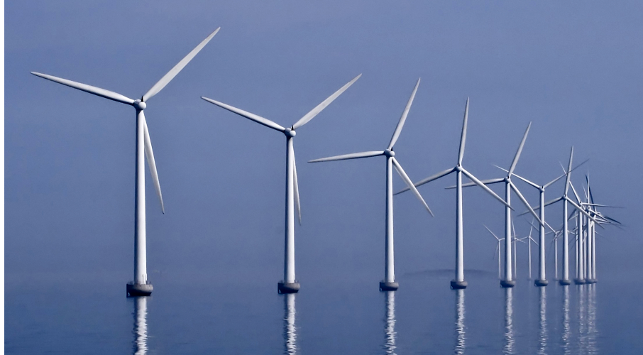
Figure 2.1: 2 MW Bonus Turbines in the Middelgrunden wind farm in Denmark [95]
