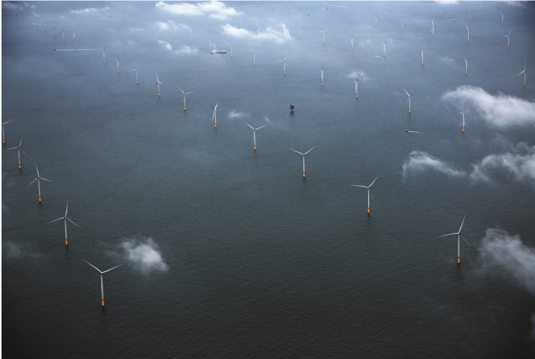
Figure 1.2: Photograph of the Siemens 3.6 MW turbines that make up the London Array off the eastern coast of the UK [86]
