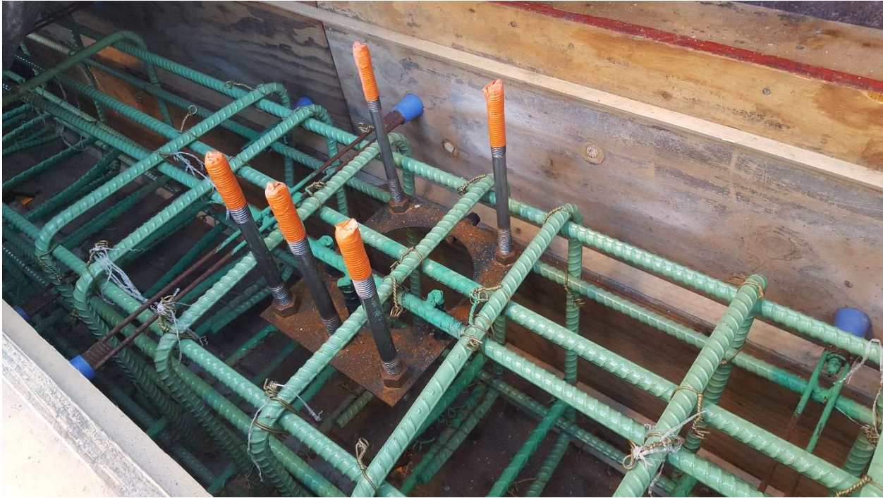
Figure 6: Guardrail anchorage and reinforcement in curb formwork. Tape on the top of the anchoring system keeps threads clean during concrete placement.
