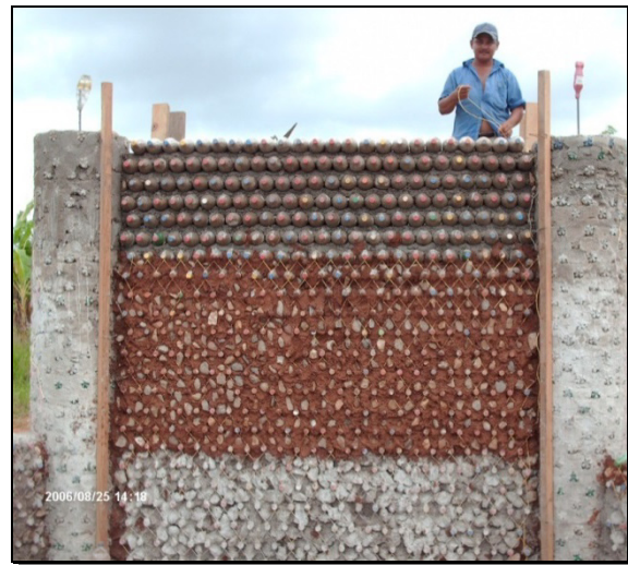
Figure 2 and 3. Building house out of plastic bottles in Honduras
