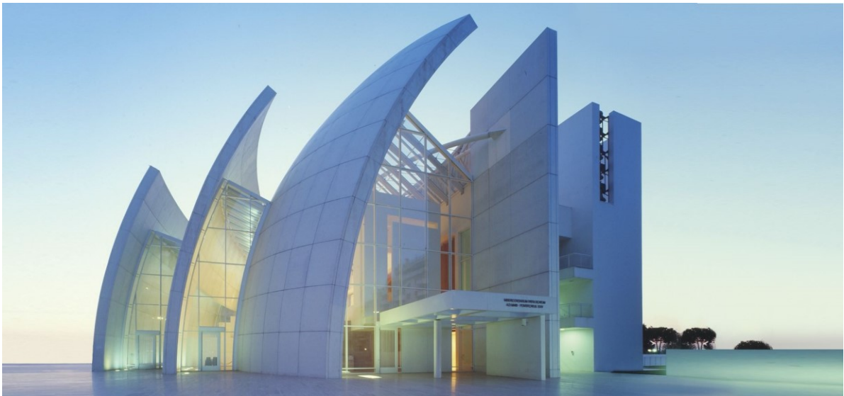
Fig. 2.6: The Dives in Misericordia , a church (in Rome, Italy) constructed of TiO 2 (Photo courtesy of Frener & Reifer).
