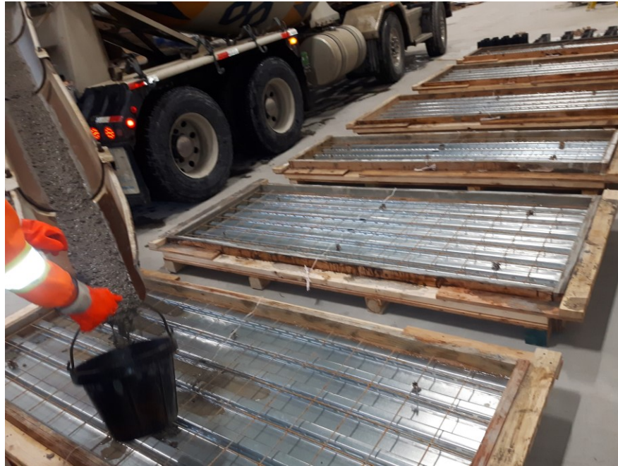
Fig. 5. Casting of high-performance concrete (HPC) slabs using a readily supplied mix
