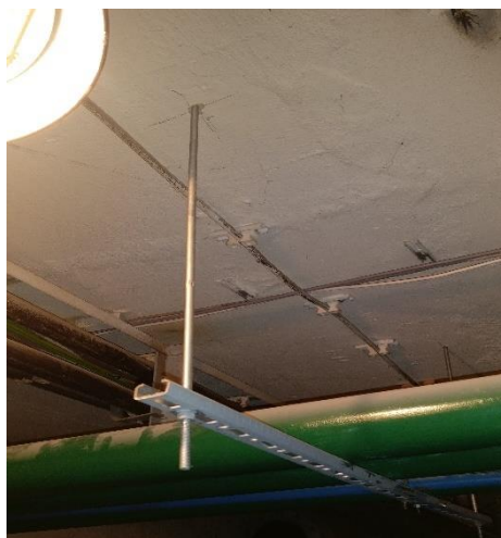
Figure 33 : Caddy clamp assembly
