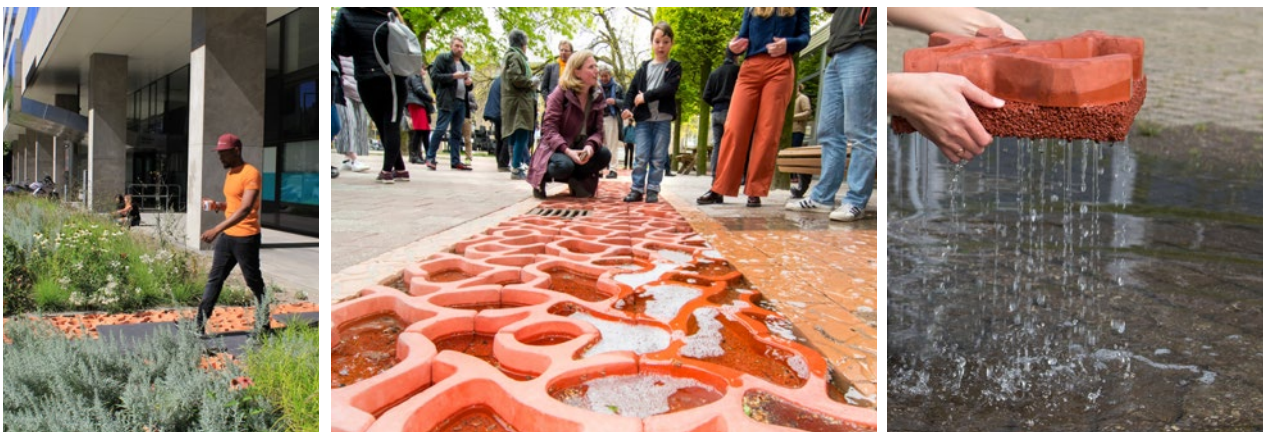
Figure 1: Rain(a)Way Katshoek Garden, Rotterdam. The “Flood Permeable” floor is composed of two different types of concrete. The lower layer is water-infiltrating and allows the rainwater to slowly seep into the ground, while the empty spaces of the upper layer accumulate water allowing users to walk freely. Source: Rain(a)Way
