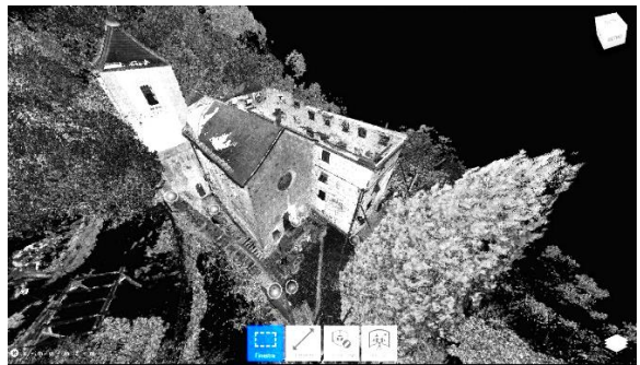
Figure 2: 3D laser scanner survey
