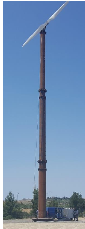
Fig. 2. PERIMA prototype with telescoping tower in its lifted position.
