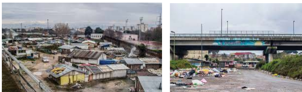
Fig. 2 Pictures of Scampia Gypsy camp. On the left, the general view of the camp is given. On the right: waste abandonment in the area surrounding the camp.
