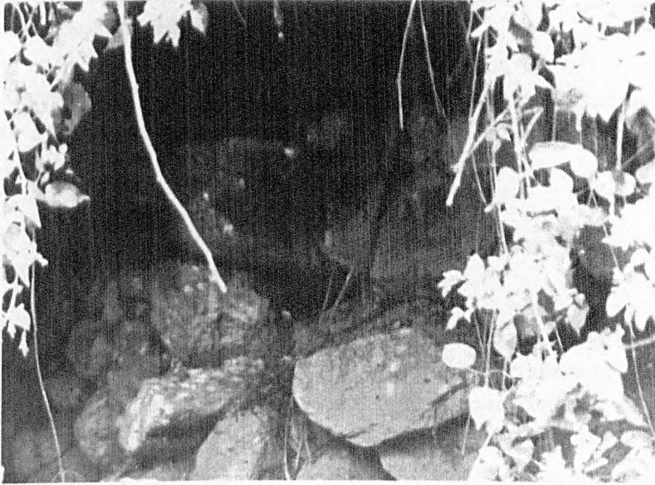
Figure 16. Typical Stone Wall
