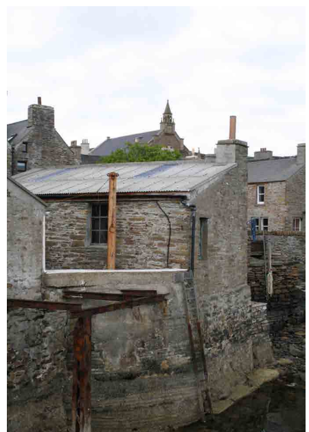
Fig 46. Pier Dundas Street
