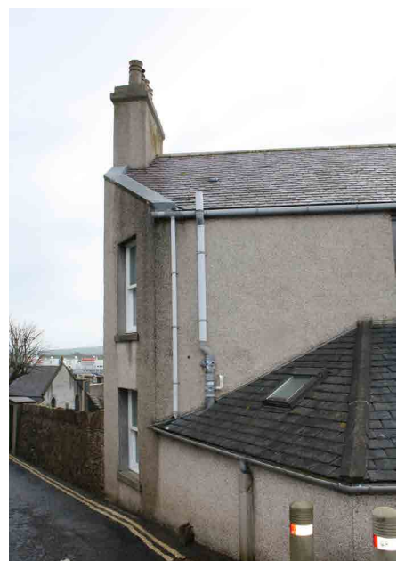
Fig 18. Church Road and Springfield Crescent
