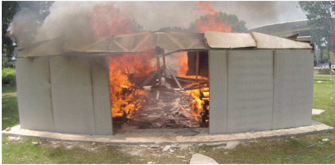
(a) Truss collapsed at 25 min 20 sec
