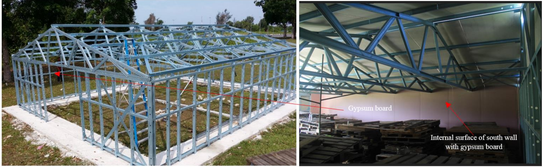
Fig. 1: Photograph of the cold-formed steel building investigated in this paper
