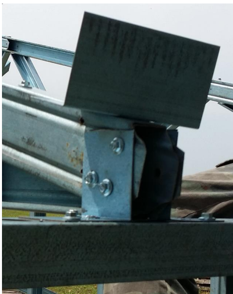
(iii) Connection between roof and top track
