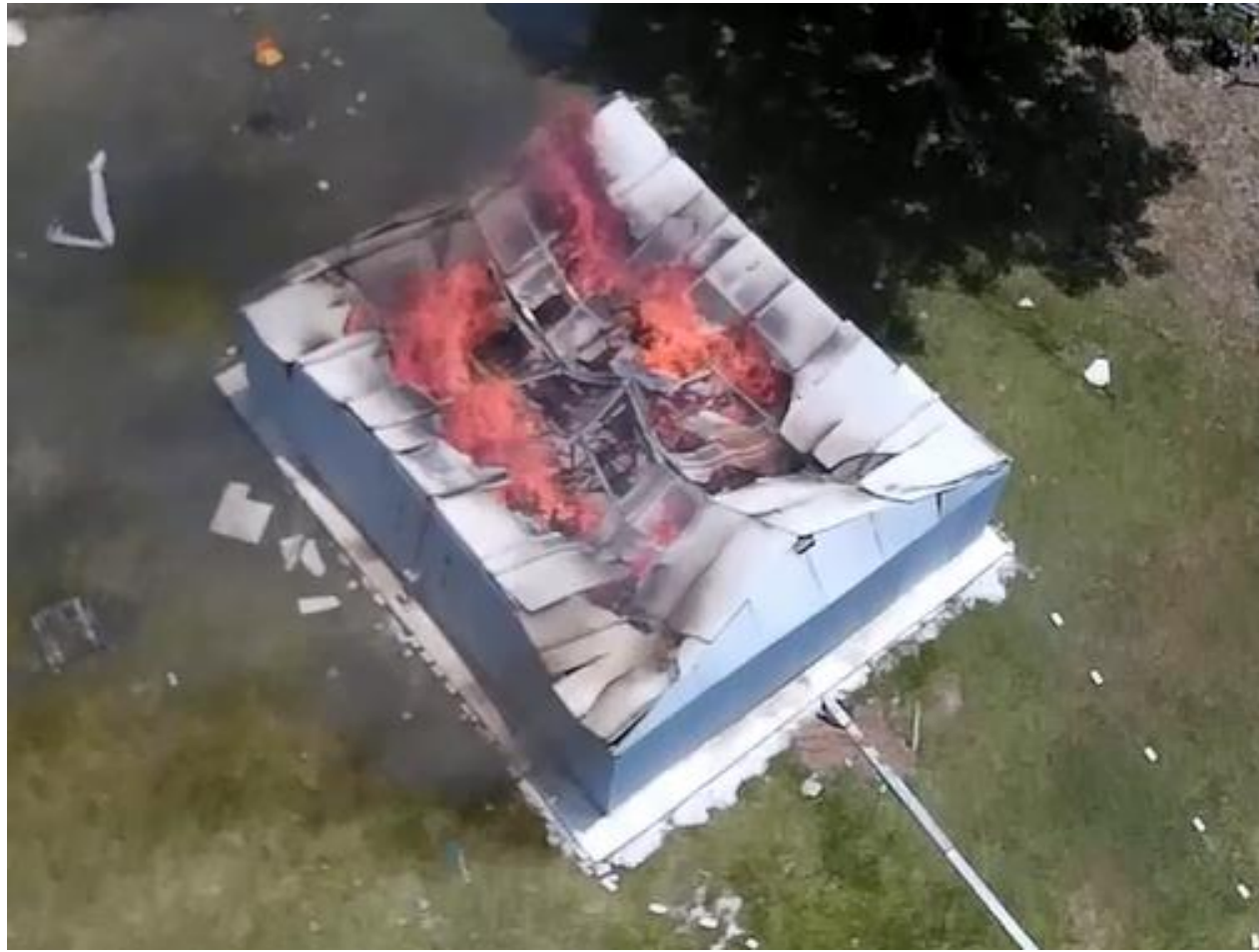
Fig. 8: Assymetrical collapse of the cold-formed steel building under fire
