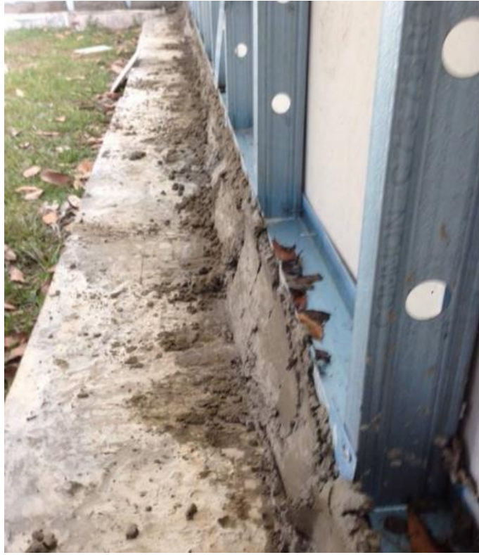
(e) Base connection after filled with concrete
