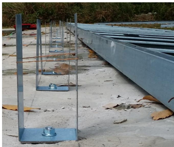
(c) Base connection of wall framings
