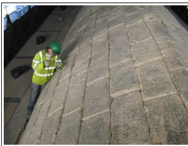
Fig. 1: Raking out vault joints.
