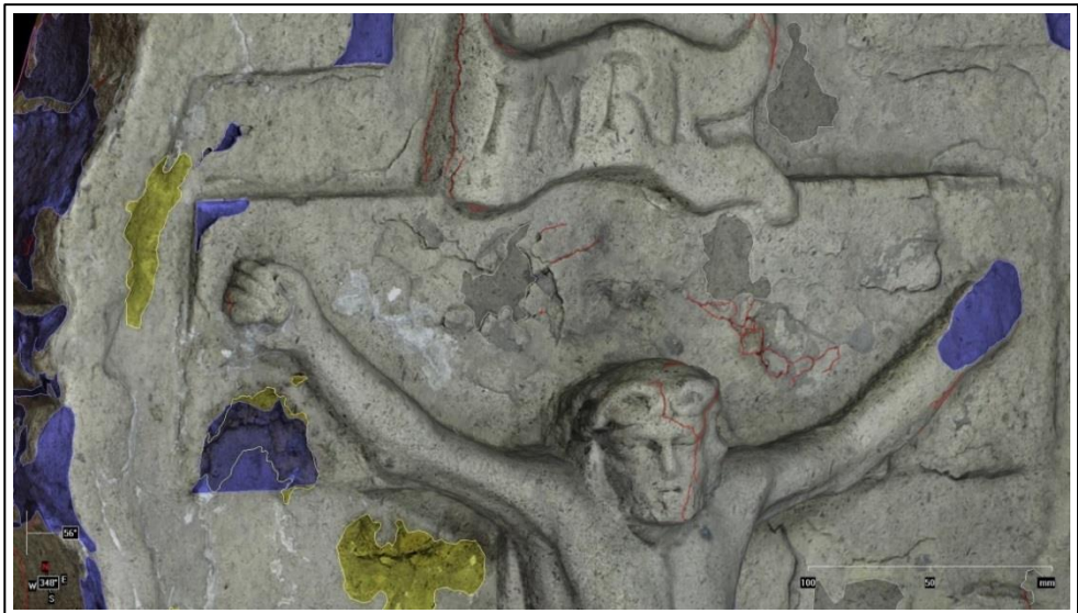
Fig. 7: 3D monument damage mapping of late baroque tombstone: Detail.
