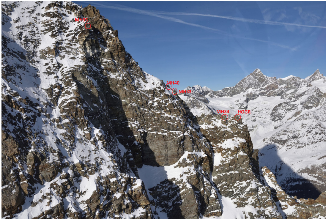
Figure C11. Winter view of the whole field site when approaching from the south. The red circles denote the GNSS measurement positions. The detachment zone is located in the shadow between positions MH33 and MH34.
