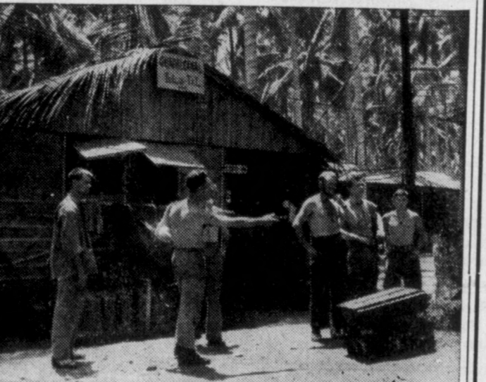
"Just getting the wire laid was a tough problem. Keeping it intact in bombings, shelling and adverse weather is a twenty-four hour proposition. . . . Wire repair crews are made up of four men. Three stand guard while the other works." (From story by Sergeant James W. Huibart, Marine Corps Combat Correspondent)
