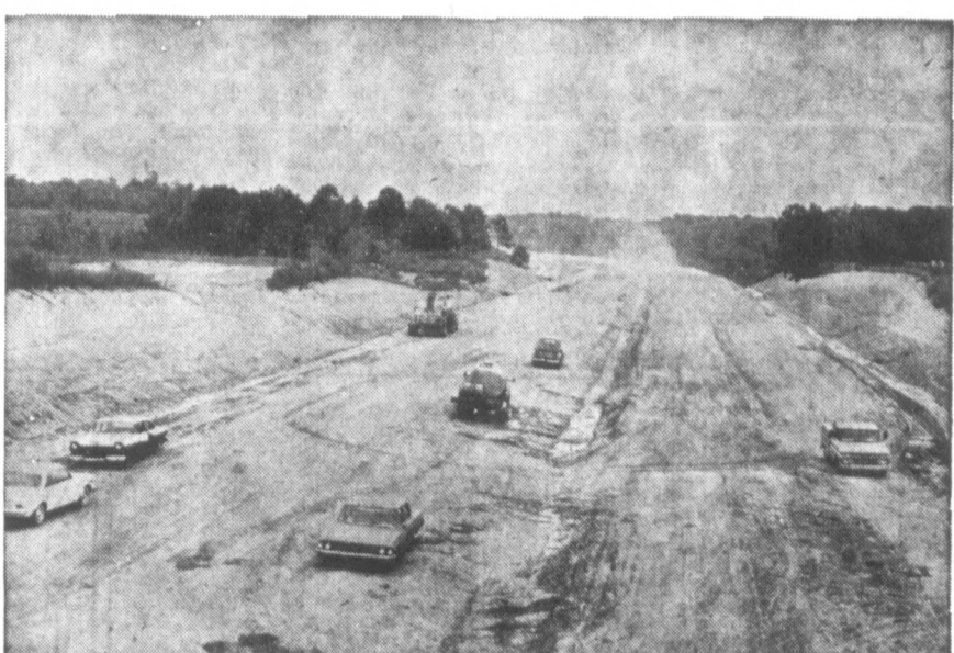
PROGRESS ON PURCHASE PARKWAY —Grade and drain on the entire 51-mile Jackson Purchase Parkway is 82 per cent complete says State Highway Commissioner Mitchell Tindler and all of the paving contracts have been awarded. This stretch of the superhighway is under construction just north of the U. S. 63 interchange in Marshall County. The route runs from the Tennessee line near Fulton to an eventual junction with I-24 between Paducah and Kentucky Dam Village State Park.
