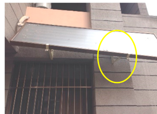
(b) Unqualified stainless-steel bracket rusts easily.
