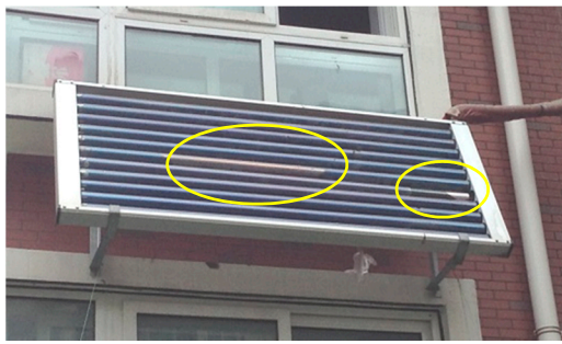
(a) Multiple broken vacuum tubes in an evacuated tubular collector with a U-shaped copper pipe inside (UPETC).
