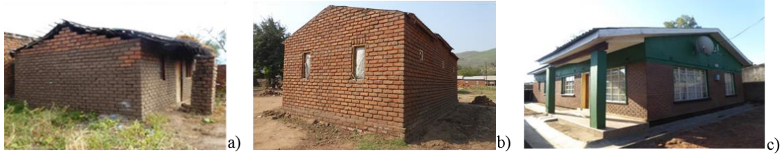
Figure 3: Typical one-story masonry building in Malawi. a) typology A; b) typology B; c) typology C
