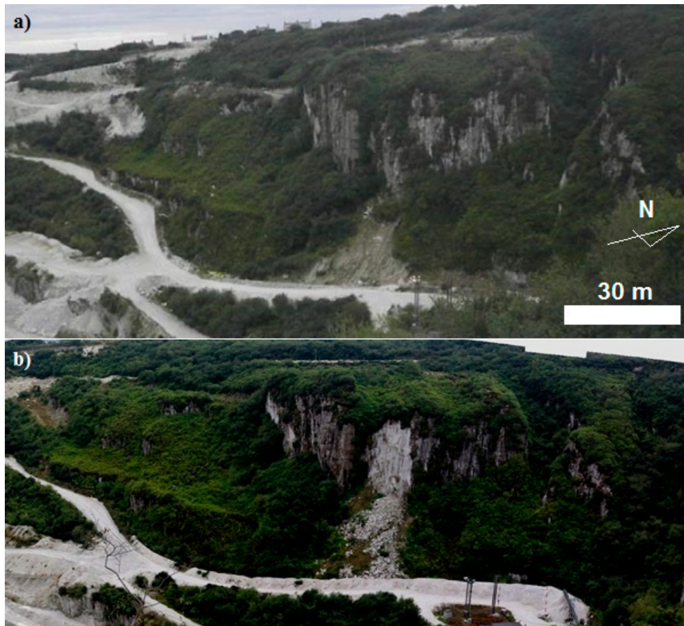
Figure 2. Photographic comparison of the rockfall (a) October 2013 and (b) August 2018. The photos were taken from the opposite side of the pit, circa 300 m away from the target and they show the change in geometry due to the major collapse occurred in early 2016. Scale bar is indicative.
