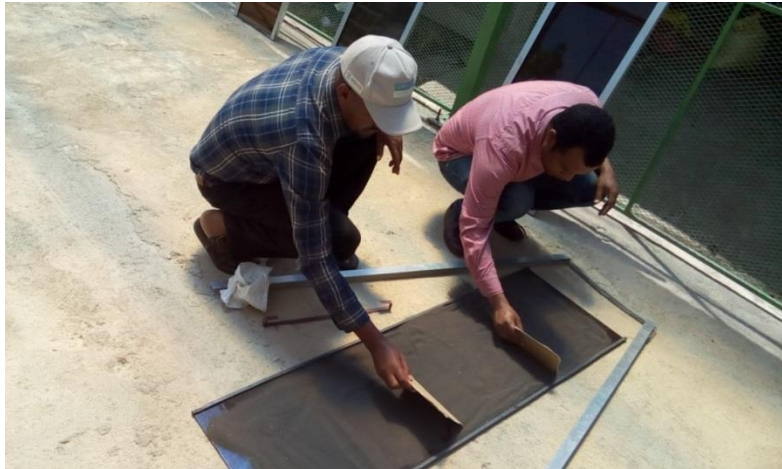
Figure 3. Sieved and blended soil uniformly loaded and spread over the dark brown PVC
