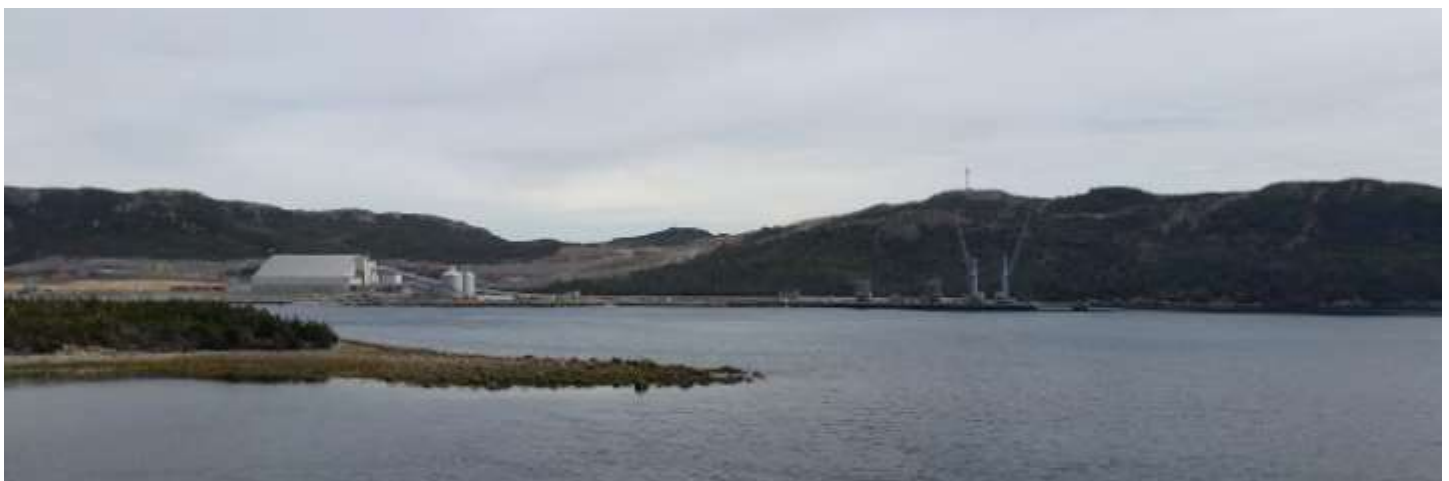
View of the nickel processing plant at Long Harbour (Photo credit: Kelly Vodden and Leanna Butters)
