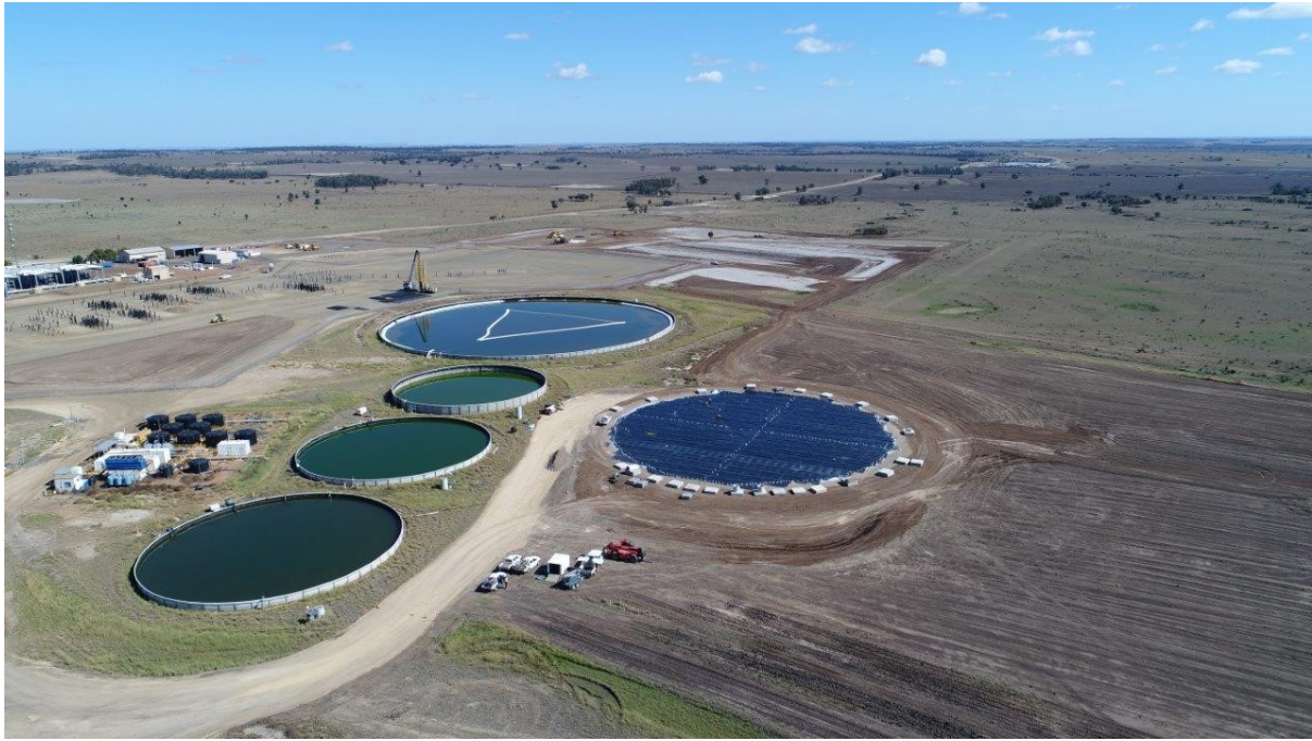
Figure 13: Modular design, concrete wall, water storage tanks utilized in the Surat Basin, Queensland, for the coal seam gas industry. Build time 9 days [61] .
