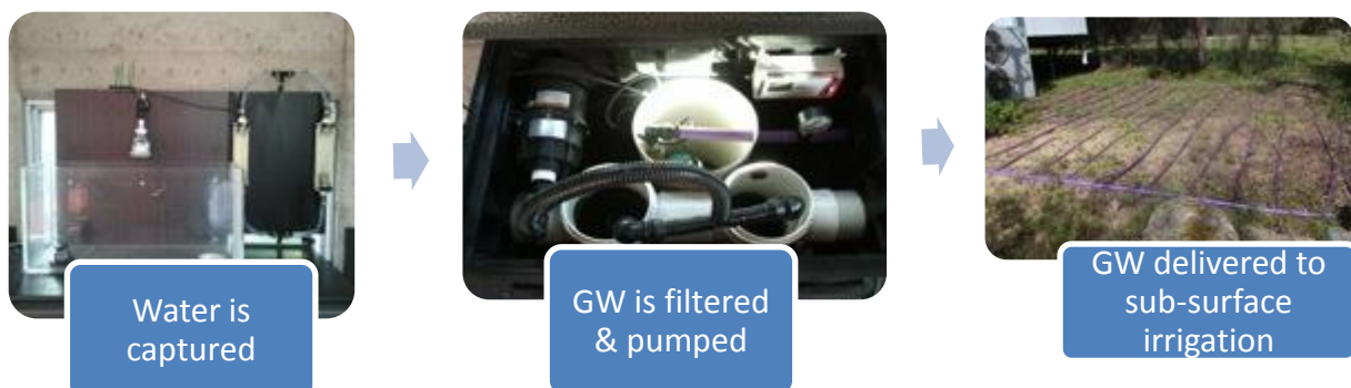
Figure 2: Greywater diversion system- general overview.
