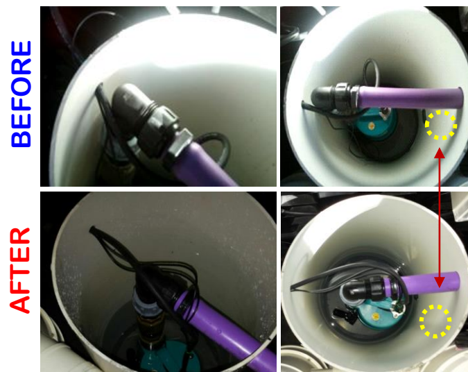
Figure 33: The pumps positioning in the surge tank, before and after.
