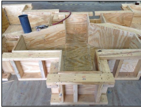
(a) Finished Forms
