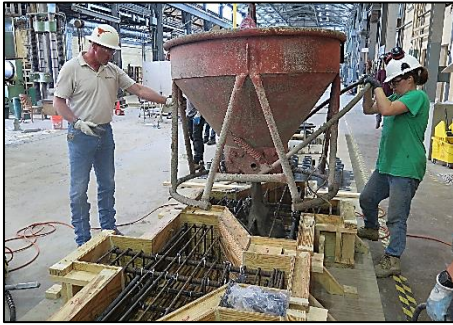
(c) Concrete Placement
