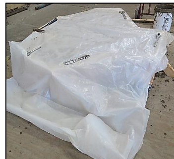
(h) Covering the Surface for Curing
