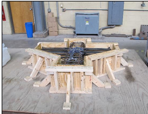
(c) Formwork for Specimen C0 (Side View)
