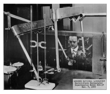
Figure 2.1: Master-Slave Mechanism for handling nuclear materials [15]
