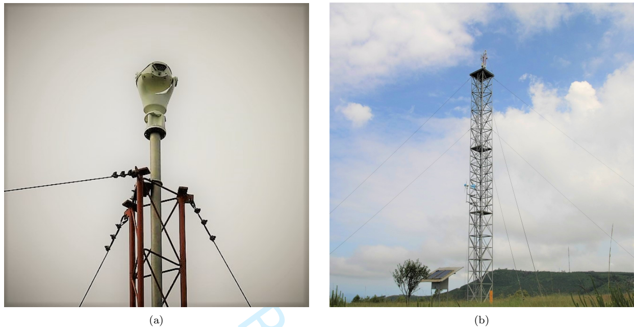
Figure 1: (a) Camera used in ForestWatch fire detection systems; (b) a 32-m tower on top of which a camera is placed, with the solar power supply visible near the base of the tower.
