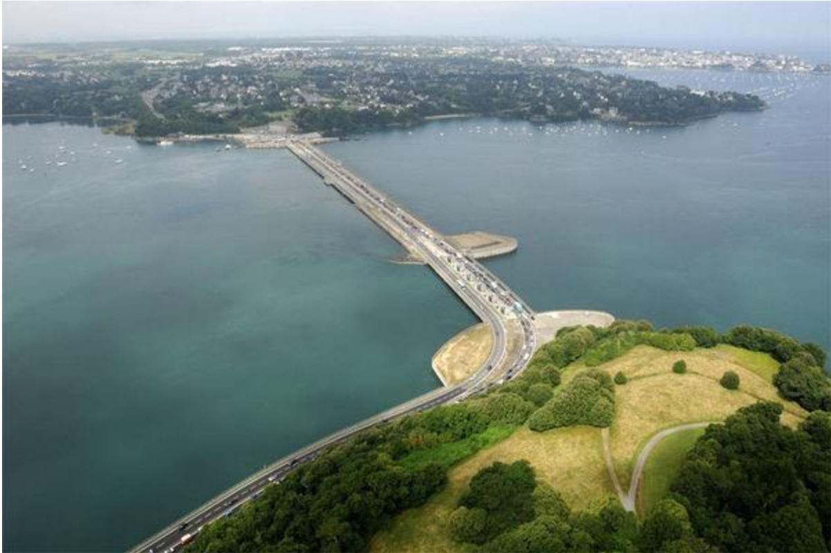
Figure 1: Photograph of La Rance tidal barrage from above (de Laleu, 2009)
