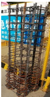
(a) Reinforcement cage
