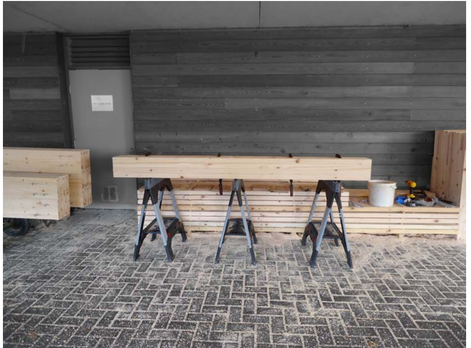
(c) Clamping of the assembled column prior to marking the bearing plate positions.
