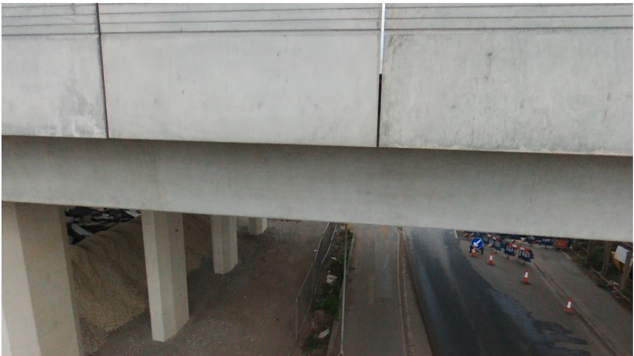
Figure 49: Snapshot of a real bridge, showing the concrete structure.
