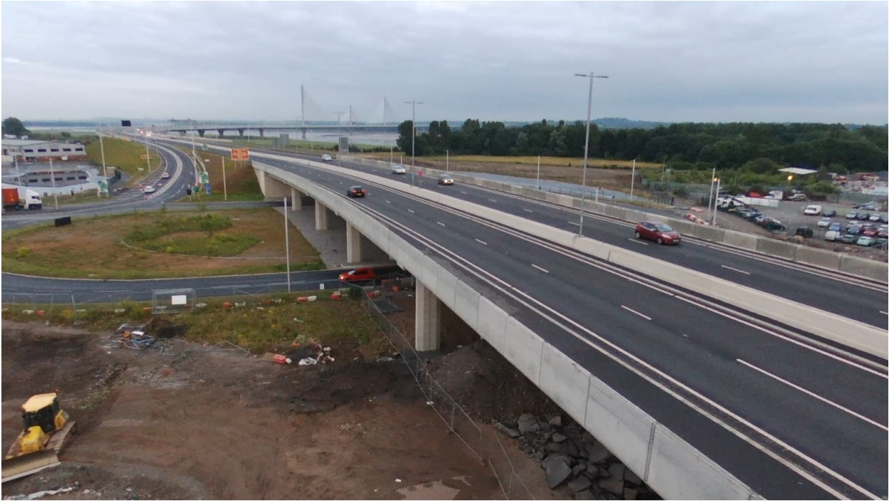
Figure 48: Snapshot of a real bridge taken by drone footage.
