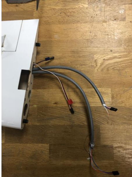
Figure 2.4 – Twisted-pair double-shielded data cabling used
