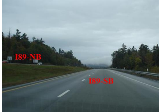
Figure 4.25. New Hampshire test site overview.
