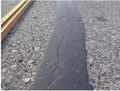
(a) Cohesive failure
