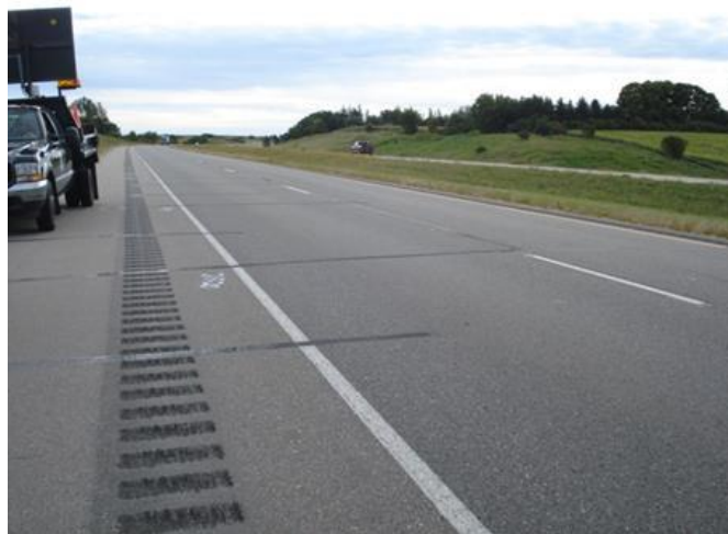
Figure 4.13. Minnesota test site overview.
