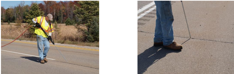
Figure 4.41. Typical cleaning operation prior to crack filling.
