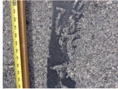
(b) Overband failure
