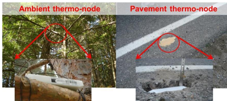
Figure 4.4. Wireless temperature nodes for ambient temperature (left) and pavement temperature (right).
