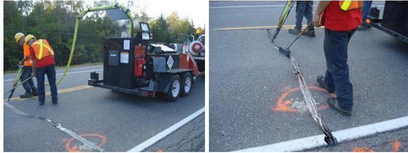
Figure 4.21. The kettle used at Ontario (left) test section and finishing with a squeegee (right).
