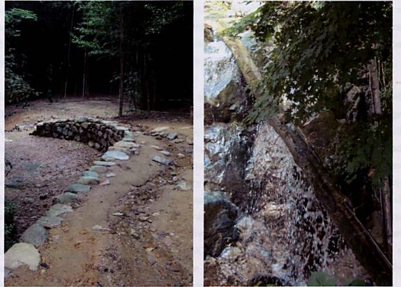
Fig. C3.9 and Fig. C3.10 Erosion of the ground and a damaged wooden gutter.
