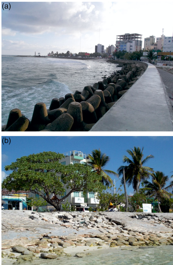
FIGURE 2 (a) The heavily engineered coast around Malé showing a sea wall protected by armour units. (b) The coastal defence structure on the eastern side of Hulhumalé
