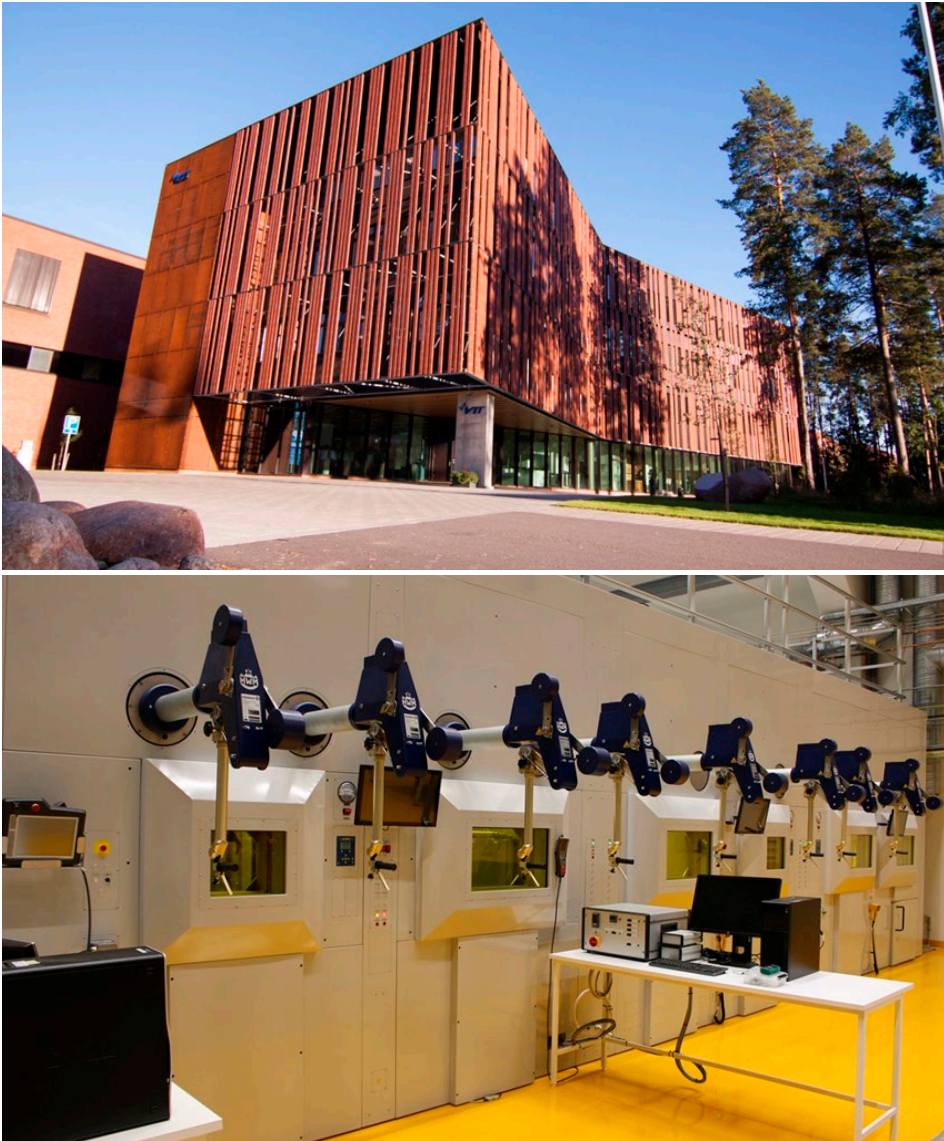
Figure 11. VTT's new Centre for Nuclear Safety (top) and the building's hot chambers for research of radioactive materials (bottom) have already been completed. Planning the waste management of VTT Centre for Nuclear Safety is important and topical. Source: VTT
